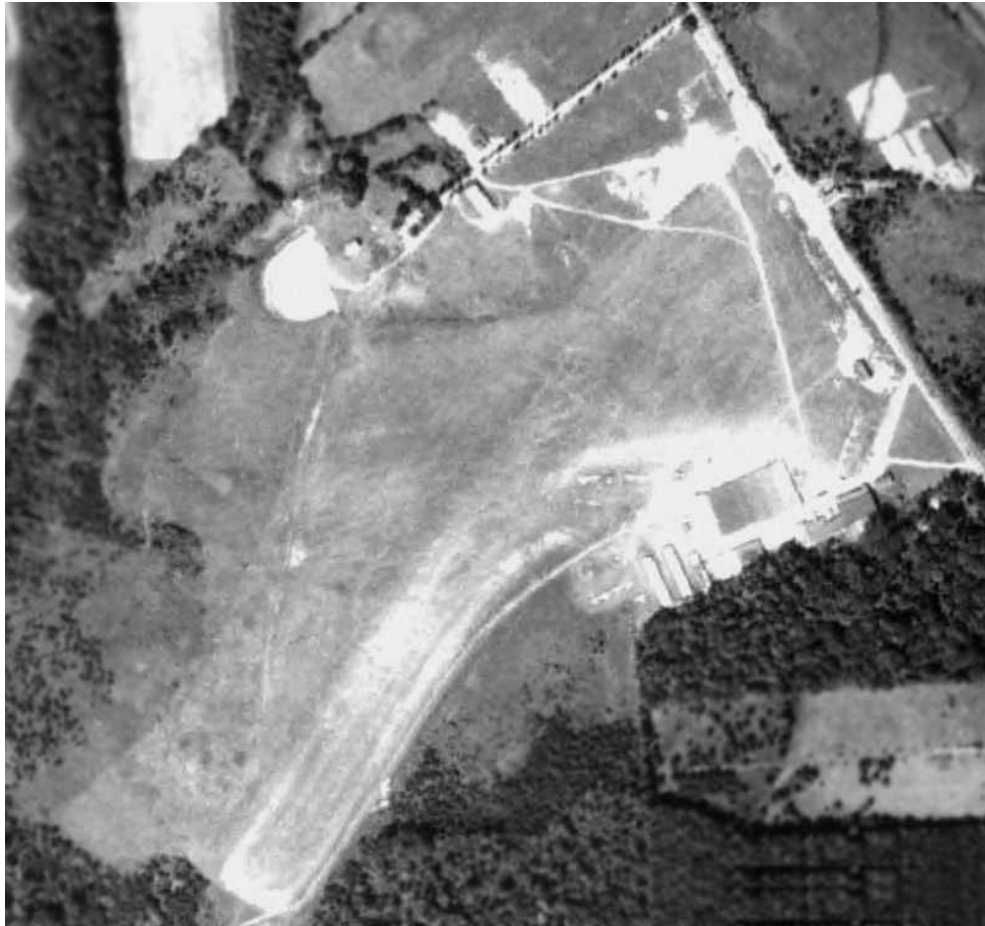
An early Fall 1951 aerial photo of Congressional Airport (courtesy of Chris Kennedy)
