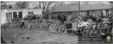
Company advertising described the motorcycle truck as maneuverable and easy to handle. It also boasted a 550 lbs cargo carrying capacity and the front mounted container provided ample space for advertising. Still, the motorcycle truck was short-lived and by 1915 it had been replaced by the easier to produce Package Truck, much to the disappointment of meat delivering services across the US.
